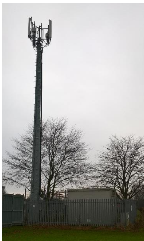
A mobile base station (the building at the bottom) with mast
