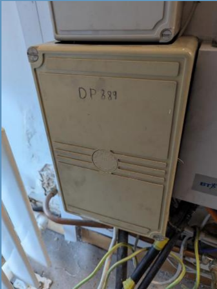
A DP (Distribution Point) with the case on
