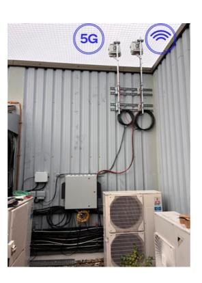
Test equipment set up for demonstrating the impact of intense use of spectrum on 5G and Wi-Fi.
